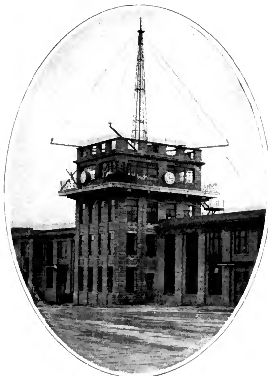
THE CONTROL TOWER
